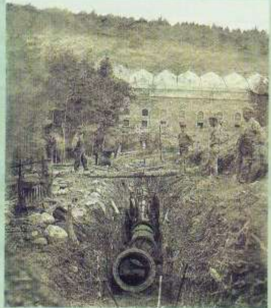
Constructing the Foyers aluminium factory, c. 1894–5.
